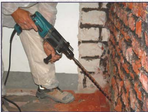
Drilling for a horizontal barrier
