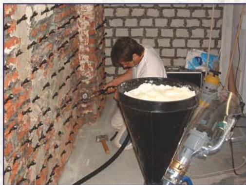
Deep injection with gel pump
